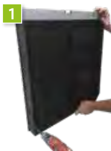
▪ Attach back frame to wall
